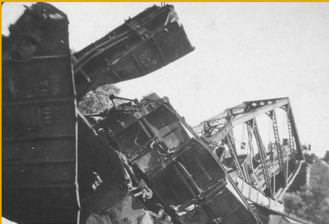
This twisted mass of steel is the result of a wreck of a Pennsylvania Railroad train as it went over the Shenango River Bridge near Clarksville, around 1917. The derailment not only destroyed the rail-cars but the bridge itself. Remarkably, crews were able to build a 580-foot temporary trestle within four days of the accident.
