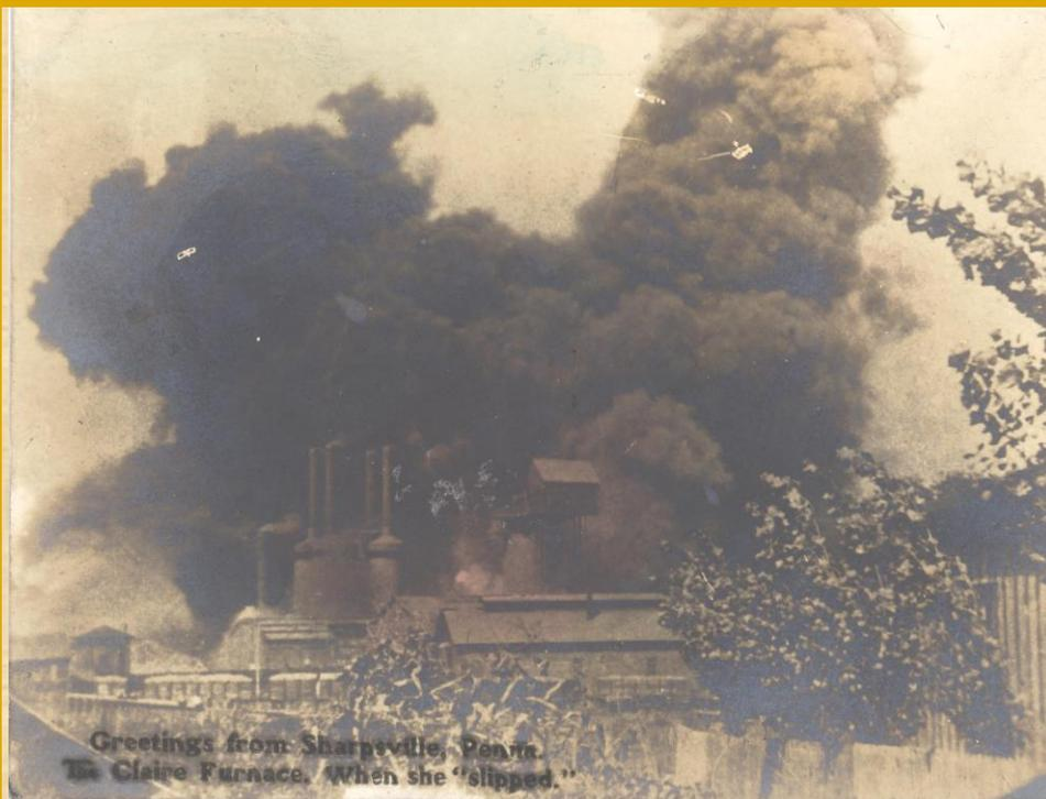
This photograph, printed on a postcard as well as in articles in the trade press, dates from July 25, 1894. The photographer had apparently set up to snap a view of the Claire Furnace, when being in the right place at the right time, he recorded the dramatic “slip”.
