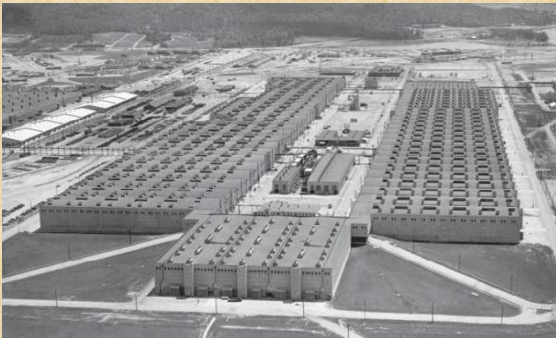
The K-25 plant at Oak Ridge, Tennessee where the Helen's research was utilized in separating the U-235 isotope in the production of the atomic bomb. When built in 1943, it was the largest building in the world.
